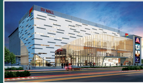
SV Mall @ Adibatla
